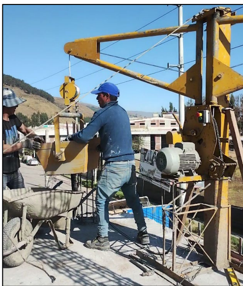
Fig. 3. Operation of an electric winch for construction.
